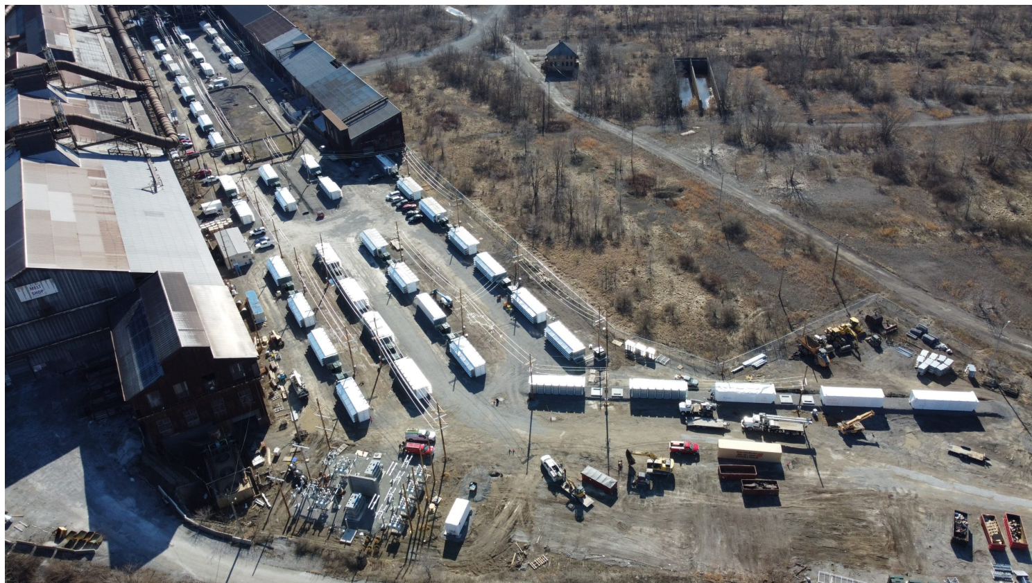
Construction underway at the Midland, PA site.
