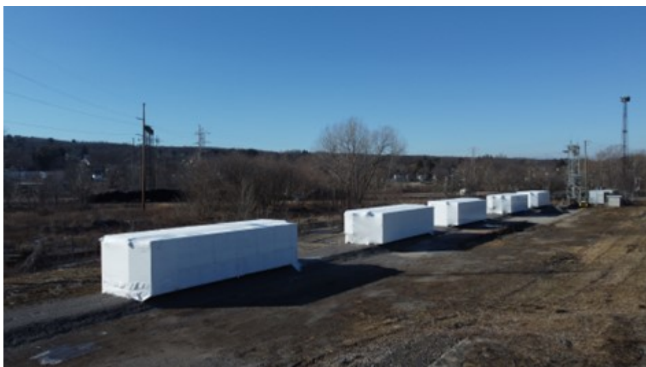
Aerial view of Sharon, Pennsylvania facility expansion
