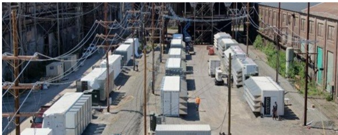
Aerial view of Midland, Pennsylvania facility expansion
