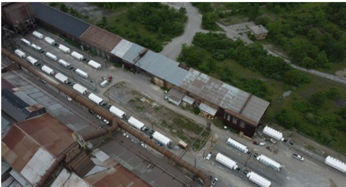
Aerial view of Midland, Pennsylvania facility expansion
