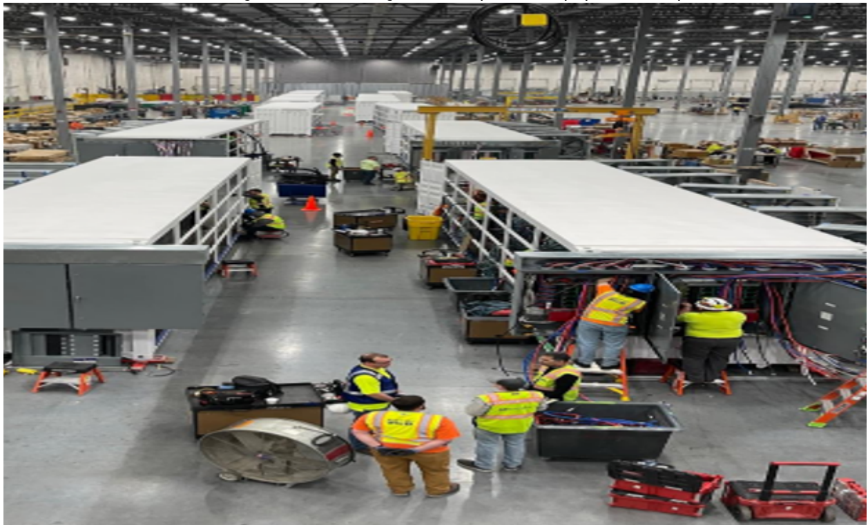
USA Modular Data Center (MDC) fabrication facility
