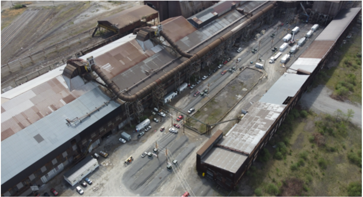
Aerial view of Midland, Pennsylvania facility development (April 2022)
