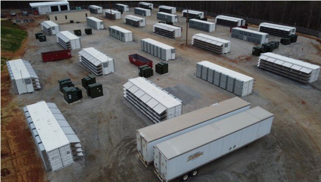
Aerial views of Sandersville, Georgia facility expansion
